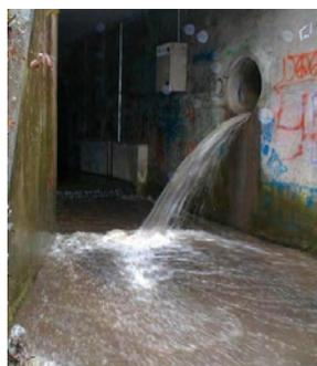
FIGURE 12: DÉVERSEMENT DIRECT AU SEIN D'UNE RIVIÈRE PÉRI-URBAINE - DÉVERSOIR D'ORAGE DE GREZIEU LA VARENNE SUR LA CHAUDANNE (69) (CREDITS PHOTO OTHU- THIERRY FOURNIER, IRSTEA)
